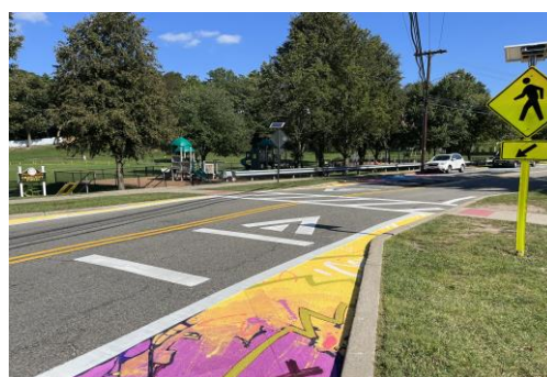
Chestnut Street midblock crosswalk after Asphalt Art Project
