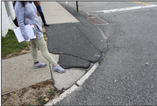
Crossing at Myers Avenue
