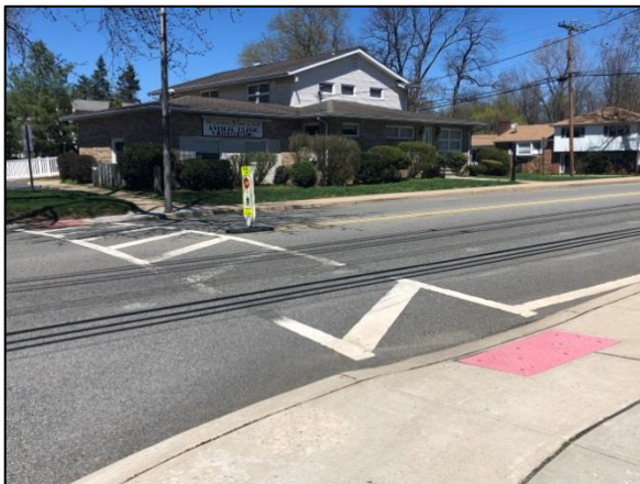
Good example of pedestrian crossing signage and truncated dome
