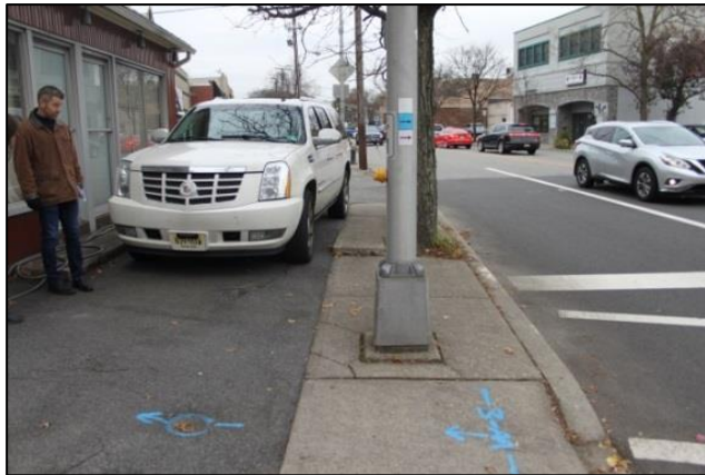
Traffic signal block that sidewalk and crosswalk at East Main Street and Bloomfield Avenue
