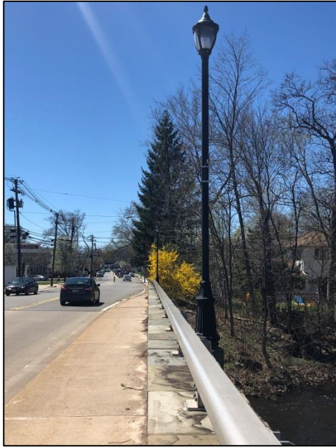
Pedestrian lighting on Diamond Spring Road
