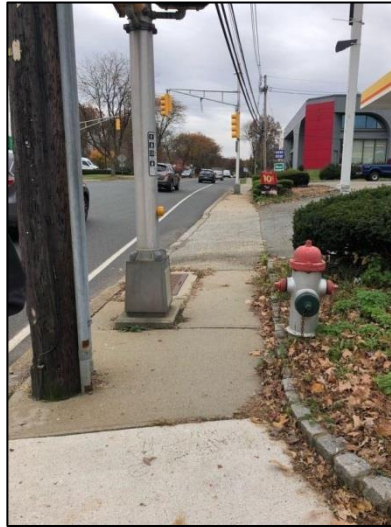
Sidewalk blocked by light and telephone pole
