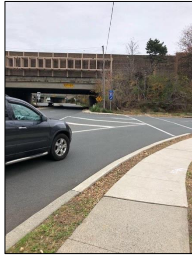
Route 80 ramp crossing is low visibility
