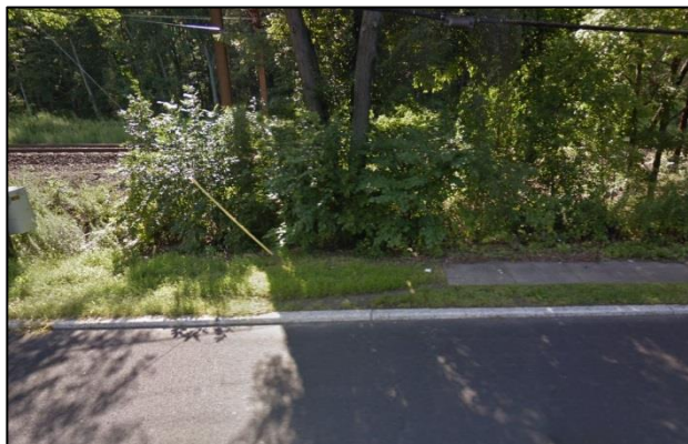
Sidewalk ends on the south side of Route 53 Source: Google
