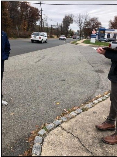
Manor Road crossing is wide, lacks crosswalk, and ADA compliance
