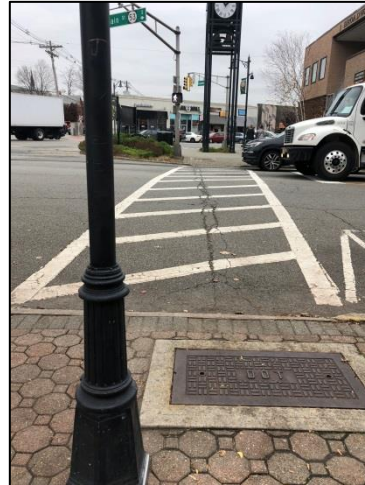
Crossing at East Main Street and Broadway
