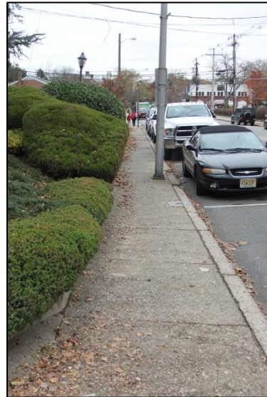
Sidewalk narrowed by post and bushes
